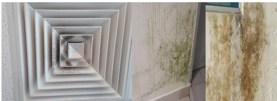
Figure 1a: Fungi growth in the duct indoor
